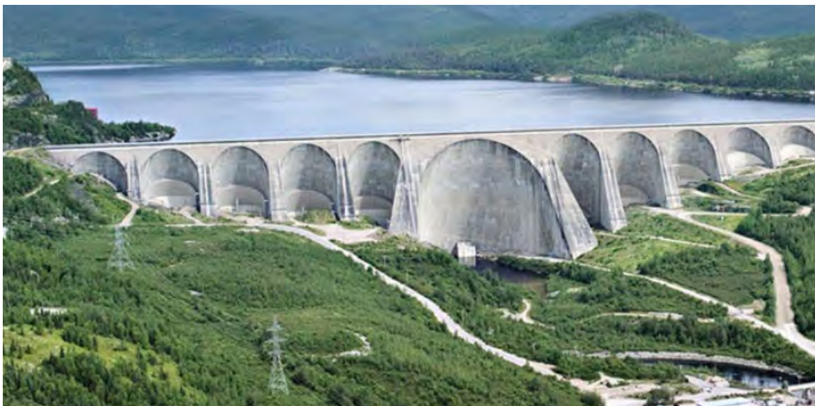
Daniel-Johnson Dam and Manic-5 Generating Station Credit: hydroquebec.com
